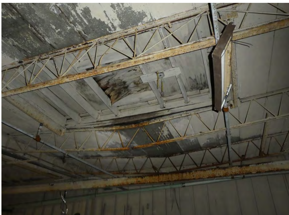
Photo 19: Building 20 presumed skylight infill, looking west.
