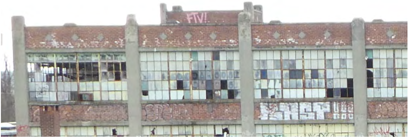
Photo 24: South elevation of Building 1. Deteriorated concrete lintels, columns, column capitals and parapet copings.
