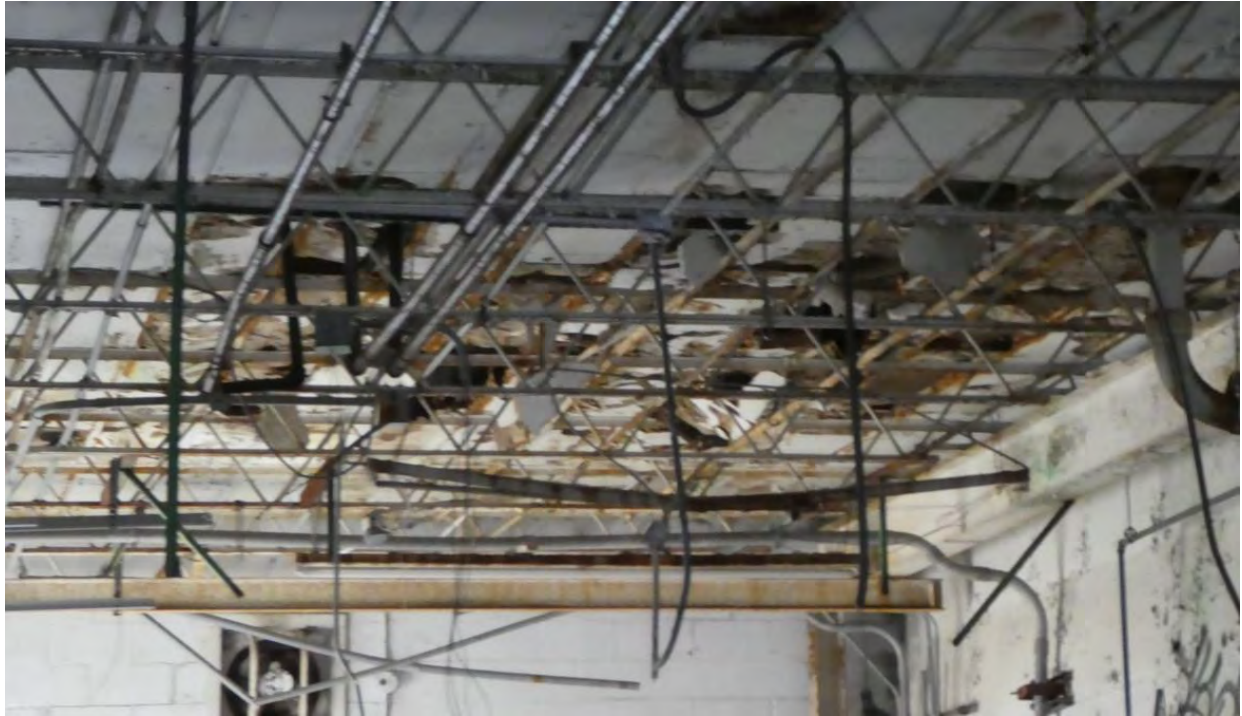
Photo 38: Building 21, gypsum plank deck failure.
