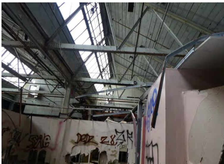
Photo 4: Building 4, looking east up at sawtooth roof.
