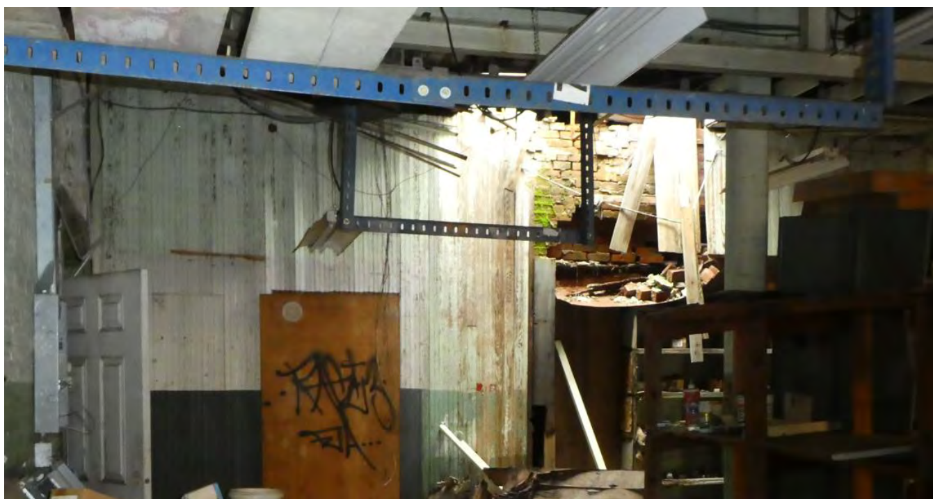
Photo 37: Building 7, wood plank deck failure.
