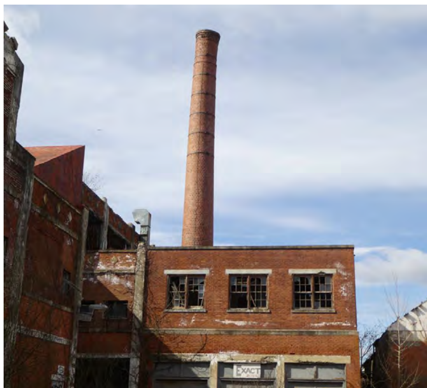
Photo 23: 98-foot-tall Boiler Flue Stack.
