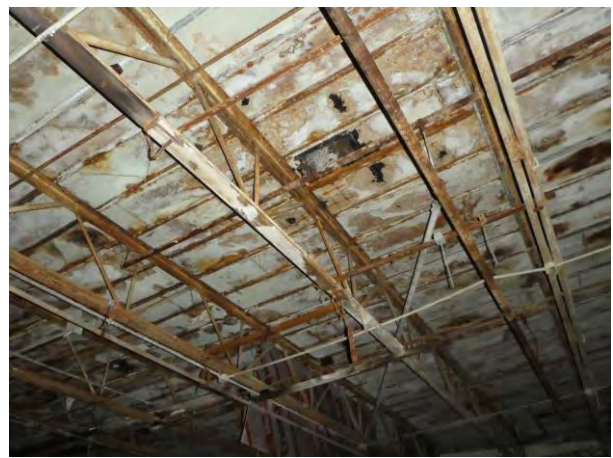
Photo 42 (left): Typical structural steel spandrel beam corrosion (Building 8); Photo 43 (right): Typical open web metal joist corrosion (Building 21).
