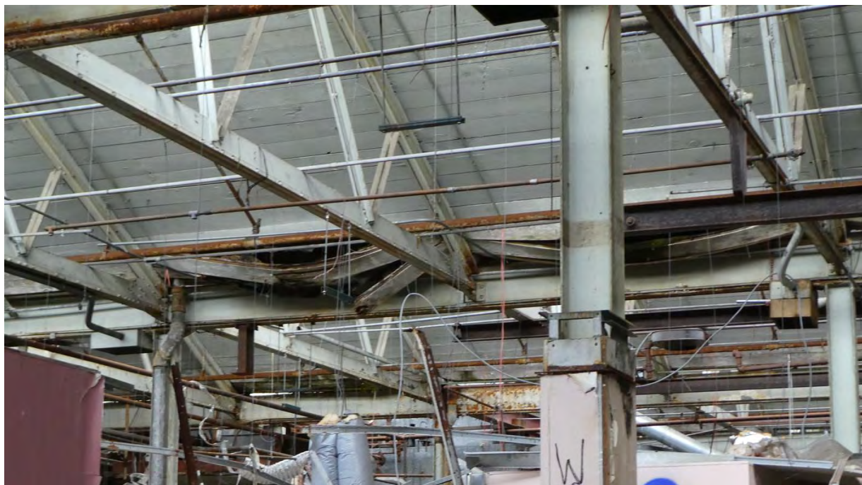
Photo 34: Building 4, wood plank deck failure.
