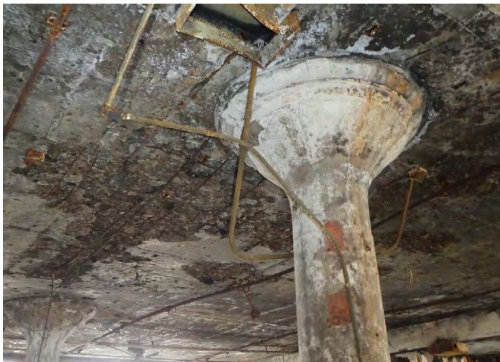
Photos 59 (above): Building 12 third floor, concentrated stored materials (looking southwest) and Photo 60 (below): Building 12 second floor looking at third floor bottom of slab, spalling, exposed rebar and sagging of slab under stored materials (looking southeast).
