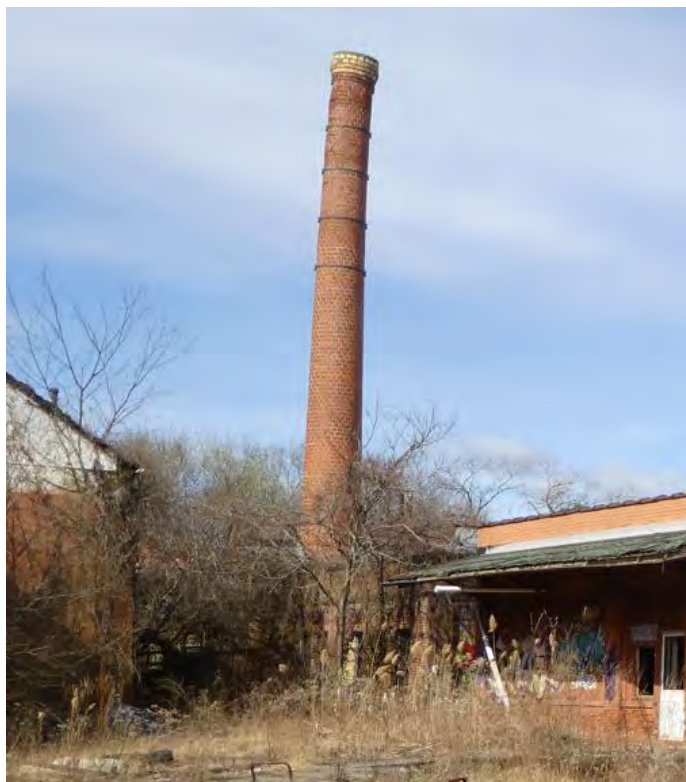
Photo 22: 75-foot-tall Boiler Flue Stack.
