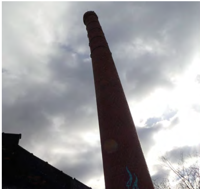
Photos 63 and 64: 74-foot-tall Boiler stack
