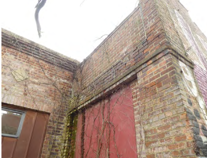
Photo 28: North Elevation Building 9. Typical occurrence of organic staining (algae, vines) and graffiti.
