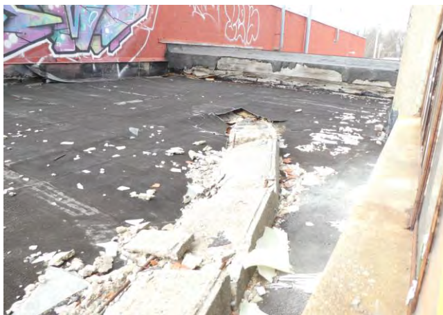
Photos 45 and 46: Lower roof west of Building 1, images of fallen coping stone and structural damage to roof deck and joists.
