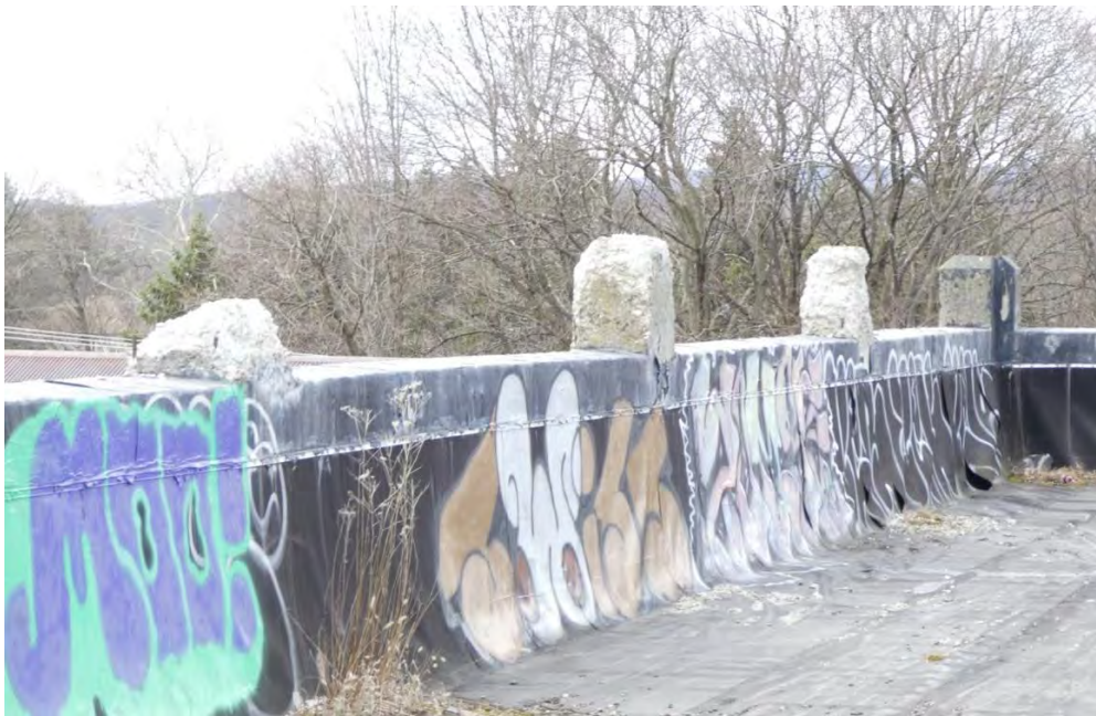
Photo 25: Building 1 South parapet wall; deteriorated column capitals.
