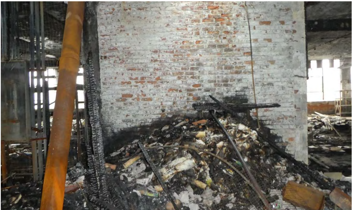
Photos 57 (above): Building 10 third floor, staining from fire damage (looking northeast) and Photo 58 (below): Building 10 third floor, building debris from fire at freight elevator (looking north).
