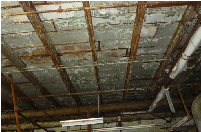
Photo 42 (left): Typical structural steel spandrel beam corrosion (Building 8); Photo 43 (right): Typical open web metal joist corrosion (Building 21).
