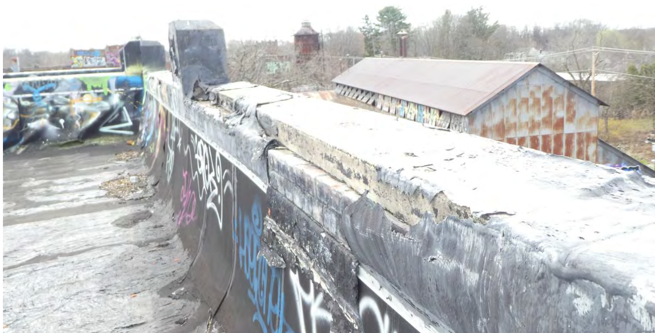
Photo 47: Building 1, west wall; coping stone at risk of falling onto lower roof.
