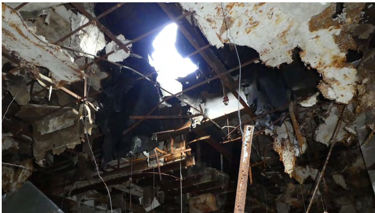
Photo 36: Building 6, poured gypsum deck failure.
