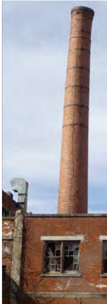
^ Existing boiler flue stacks
