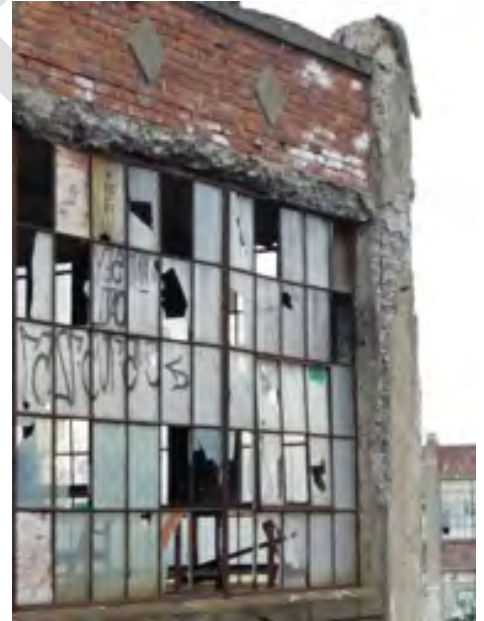
^ Existing exterior walls and windows
