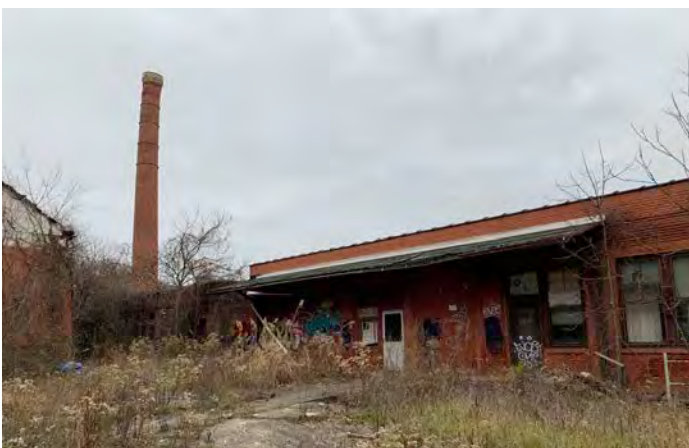
6 Dilapidated 1926 South Factory building with smokestack
