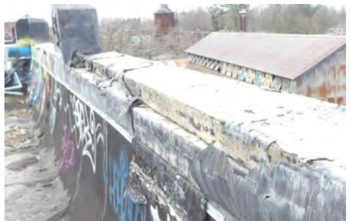
^ Existing condition rooftop parapet coping
