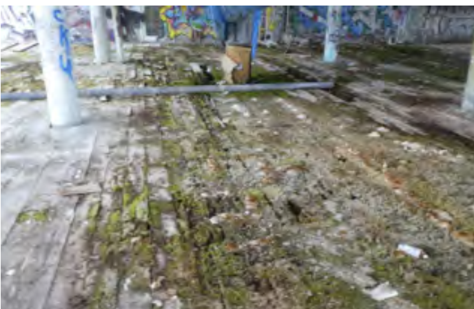
^ Existing floor condition
