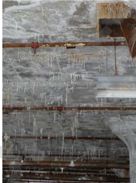
^ Existing roof condition
