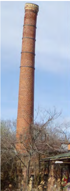
^ Existing boiler flue stacks
