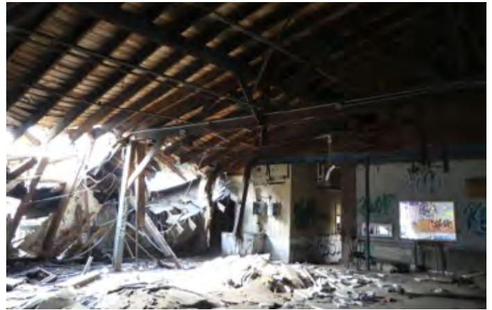
^ Roof collapse
