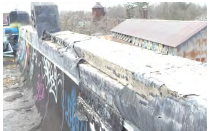
^ Existing condition rooftop parapet coping
