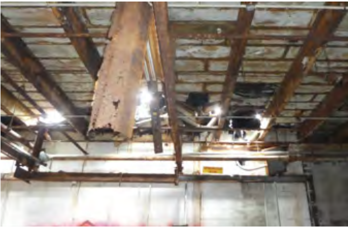
^ Roof collapse
